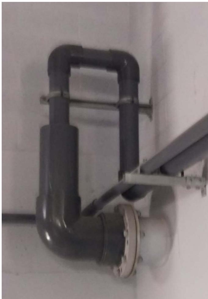
Figure B.1.2 Air gap on the potable water top-up at the entry to the recycled water storage tank is clear of any wrapping.
