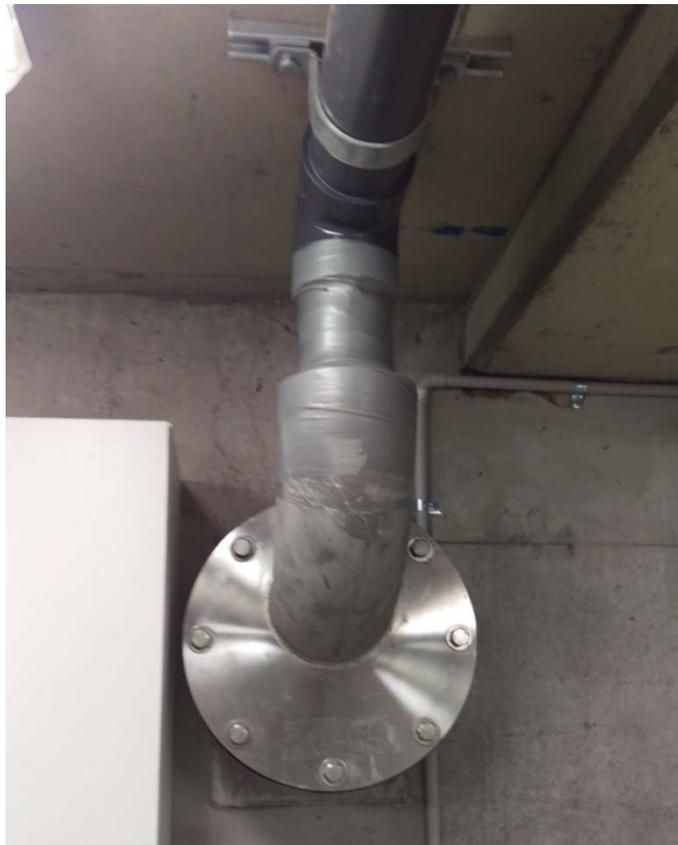
Figure B.1.2 Air gap on the potable water top-up at the entry to the recycled water storage tank remains taped.
