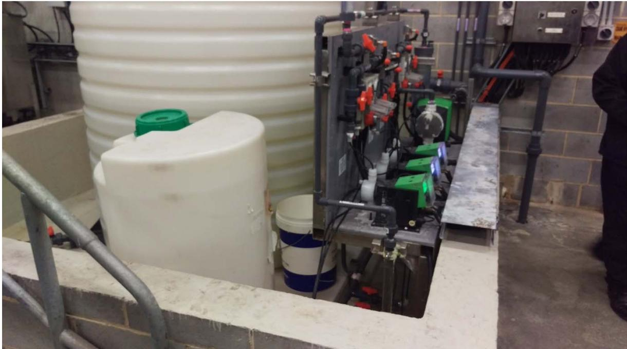
Figure A.3.1 Plastic container located within chemical storage bund.
